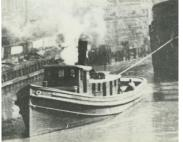
Rand & Burger, Manitowoc, WI, built a wooden towboat for C. M. Charniey, Chicago. Her measures were: 78'4" x 19' 1" x 9' 1"; tonnage 83.98 grt, 41.98 net. She was powered by a high pressure non-condensing engine, 25" x 26", built by Cuyahoga Iron Works, Cleveland.She was assigned official number 126117.
