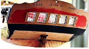
Windows installed on the stern and side galleries
